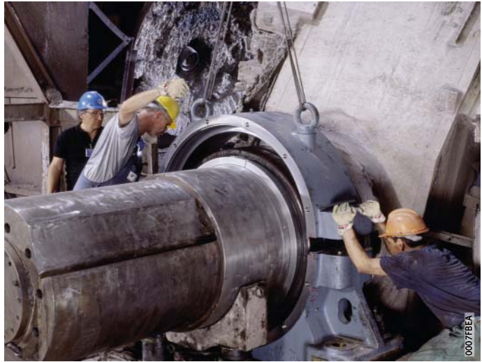
Figure 1 Mounting service on a converter
